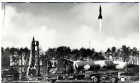
The 14m V-2 rocket is propelled by alcohol & liquid oxygen fuel to an altitude of 90km at a speed of 5400km/h with a range of 320 km & a 740 kg load. All modern rockets including the Saturn V moon rocket are based on the A4 concept.
