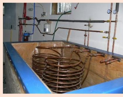
was put up against that. Then I epoxied the whole thing including multiple layers in the corners. I thought that I could use the tank like that, but the heated water softened the epoxy and eventually parted and leaked at the seams. So I added a high temp liner made by a liner company out west. This works well and can handle temps of 200 F or
