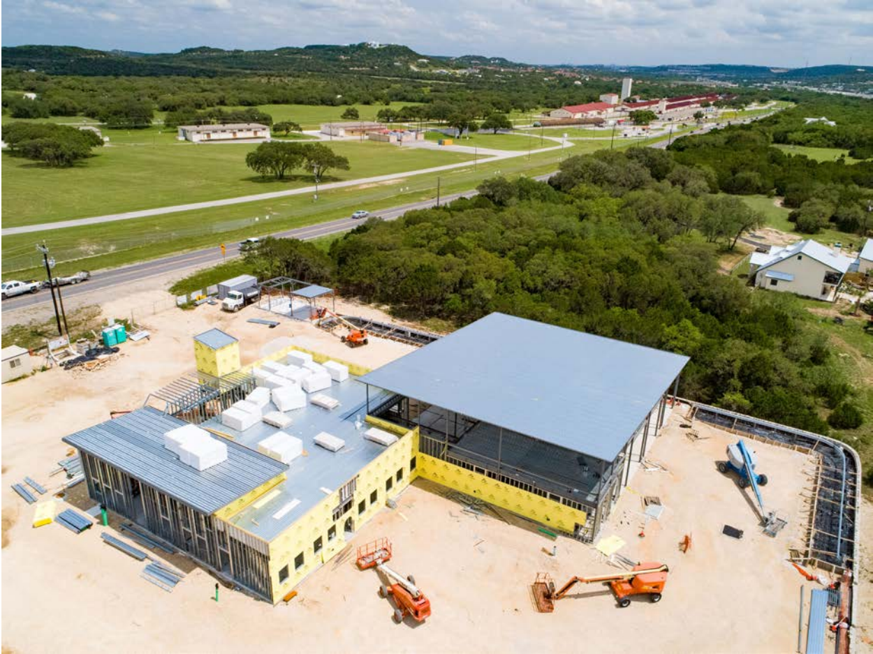
EXHIBIT 1 – FACILITY FOOTPRINT – SLAB & STEEL ERECTION 05.31.21
