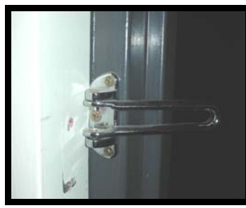
Figure 4 – Example of Security Device which, if activated whilst the door was open, would prevent the door from latching.
