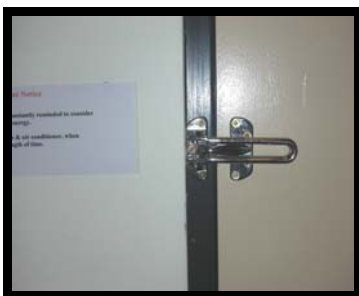
Figure 4 – Example of Security Device which, if activated whilst the door was open, would prevent the door from latching.
