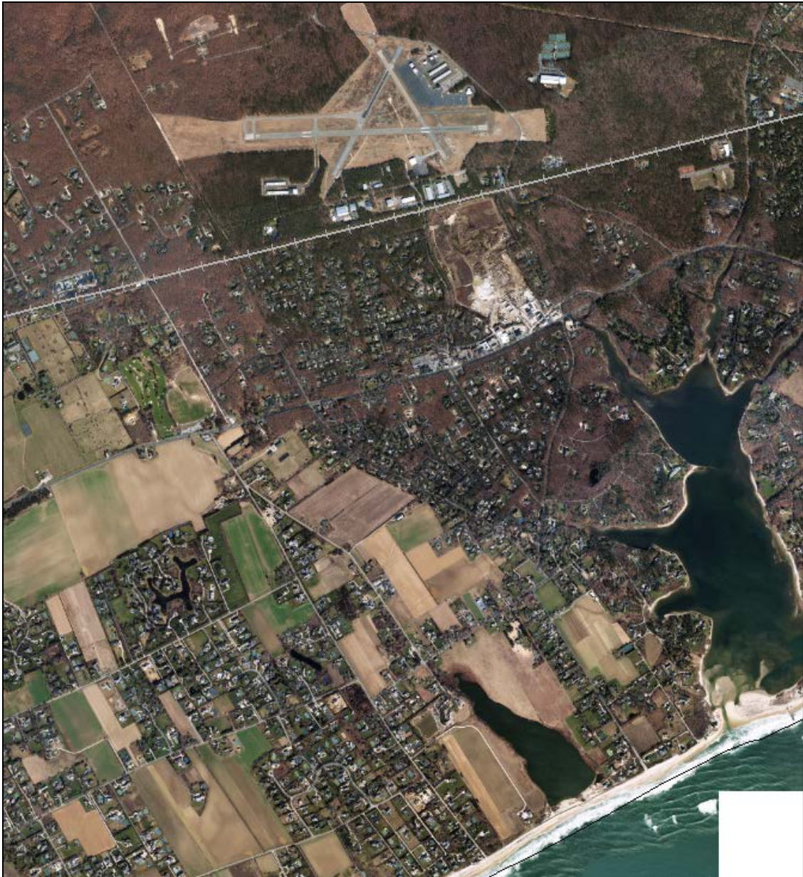
Figure 4 Aerial of the Immediate Vicinity of the Proposed Main Installation
