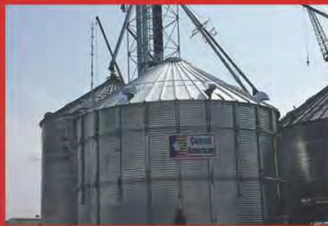
Grain Bin Construction and Remodeling
