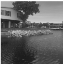
Rip Rap Seawall
