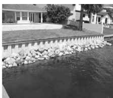
Vinyl Seawall with Rip Rap
