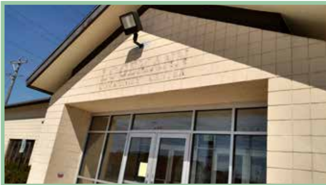
The Logemann Community Center ceased operations at the end of 2015.
