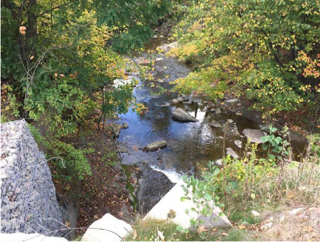
Figure 53. Elk Creek crossing under Oliver Road, steep-sided gorge; bridge supported by gabions.
