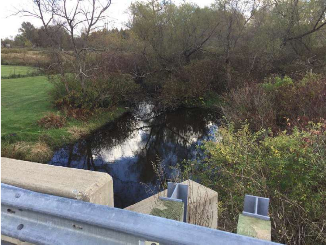
Figure 51. Elk Creek, looking downstream at Greenlee Road bridge, northwest of the Marsh Site.
