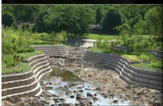
Storm Water - Incorporate Redi-Rock's 9 In. Setback solution for storm water applications and to build even taller gravity walls. 9 In. Setback walls look great, increase a channel's volume, and also create safer, more gradual slopes.
