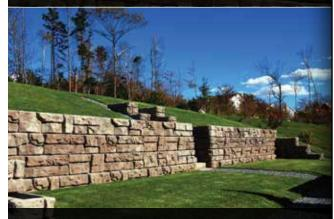
Gravity - Massive, one-ton Redi-Rock blocks rely on gravity to hold back slopes in many different applications, including this Ledgestone wall. Even taller reinforced walls are possible; visit www.redi-rock.com for more details.
