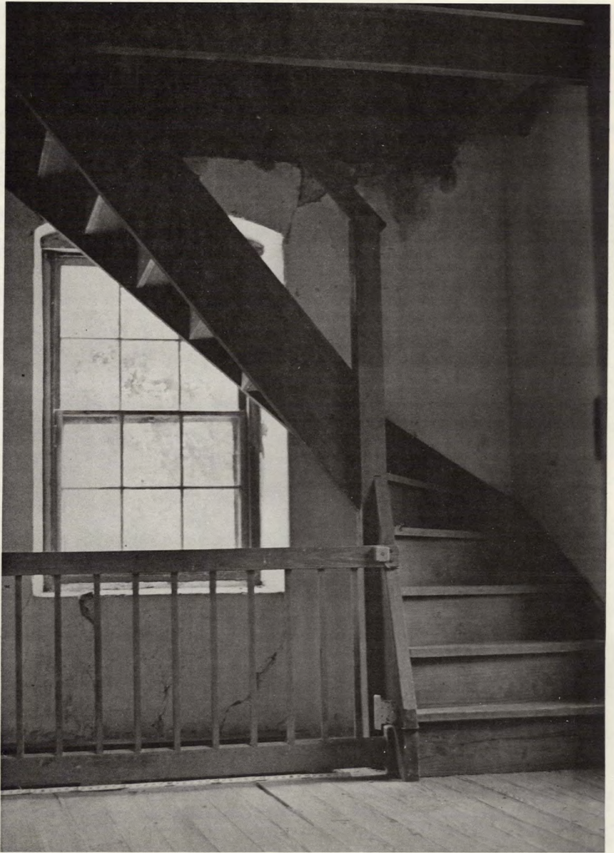
Figure 11. Interior Stairs, Second Floor.
