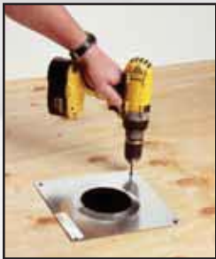
Mount SureGrip support plate.
