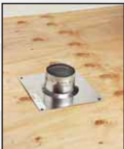
Push pipe through vent support.
