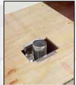
Push pipe through vent support.
