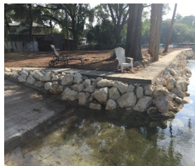
Native Limestone Boulders-Rip Rap
