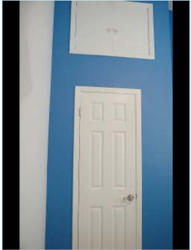
additional storage above closet
