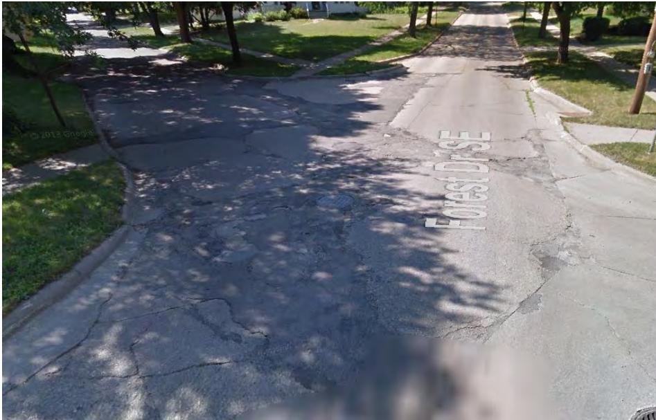
Figure 9: Perhaps the worst location in the City, an entire intersection with PCI < 10.
