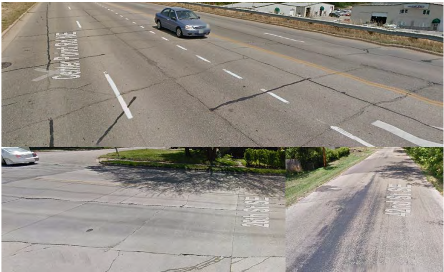
Figure 7: Example of Fair road condition.
