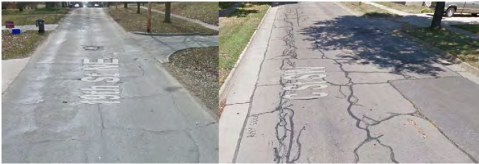
Figure 8: Example of Poor road condition.
