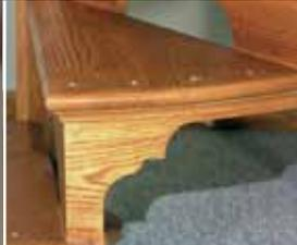
The miter returned end of each tread is finished with a decorative trim bracket and cove moulding which are curved to match the radius of the spiral stairway.
