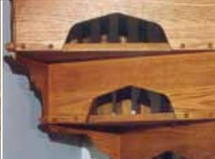
The underside of the treads and risers provide a clean, finished look. Note: the riser cutout design rejects a 4" sphere ball.
