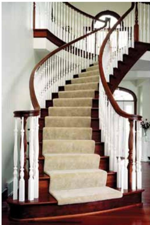
**Bending rails are typically used on circular or spiral stairs, and curved balconies.**
