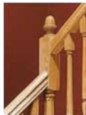
Handrail runs straight into the top block of the newel post at all landings.
