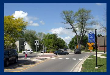
**Pedestrian Enhancements:** There are a large number of improvements that can be made to help protect the pedestrian. Intersections can be improved with count-down signals, signage can be improved, and paint markings can define pedestrian space across an intersection. Refuge islands can be constructed across busy corridors to provide a safe stopping point for pedestrian safety.
