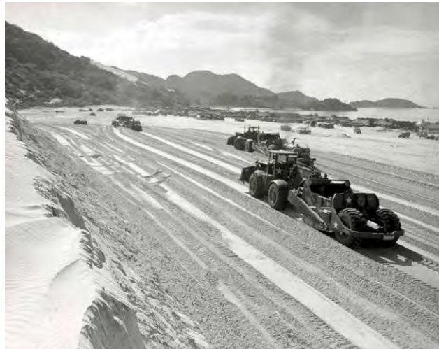
84 th Engineer Battalion provided early construction at Cam Ranh Bay, 1965
