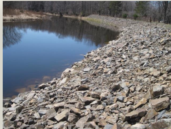
Rock rip-rap treatment for shoreline erosion
