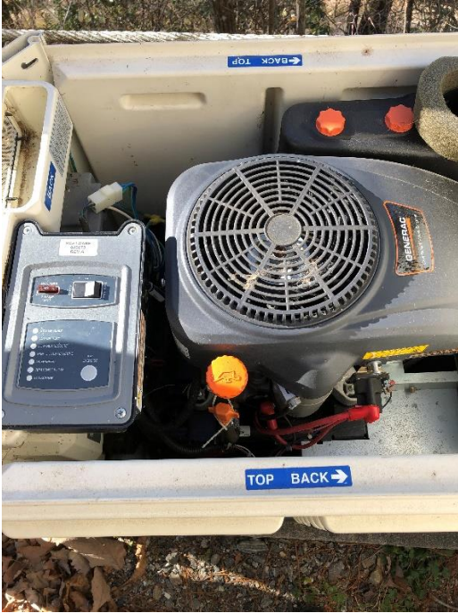
Image: North Tank House Generator – Top Removed
