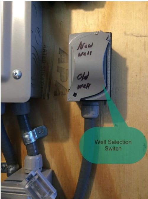
Image: North Well Control House Well Selector Switch
