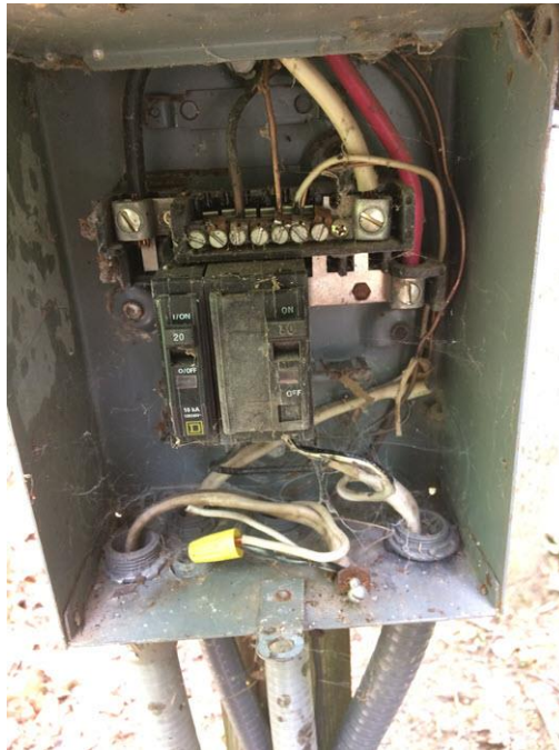
Image: Power Into the Crossover (The older conduit is the signal wire from the North Tank)
