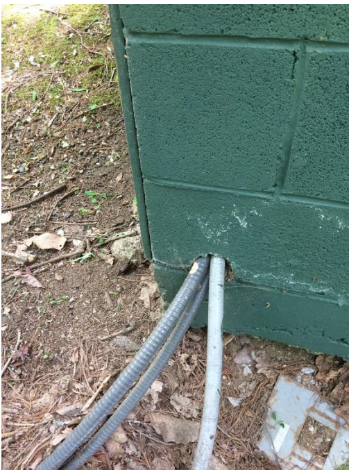
Image: Power Into the Crossover (The older conduit is the signal wire from the North Tank)
