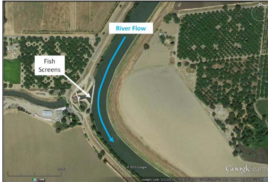
Figure 5. Aerial photograph of an example of an existing Sacramento River flat-plate fish screen located on an outside river bend to maintain high sweeping velocities. Water velocities passing the screen typically range between 2 to 4 feet/second (USBR 2006).
