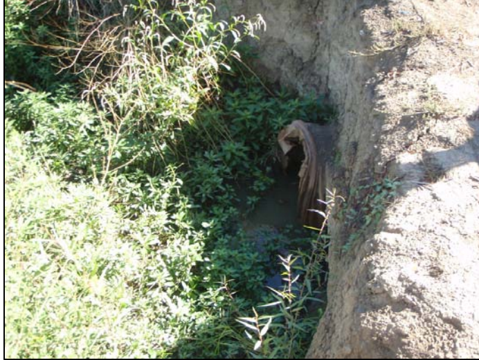
Figure 26. A culvert and unimproved road crossing in the Tule Canal. Photo by Dave Vogel.
