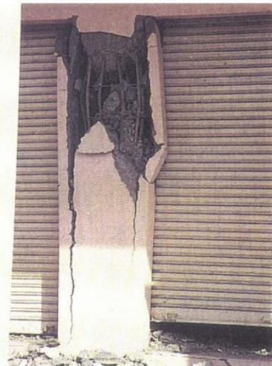
Figure 1.2 cracking in columns
