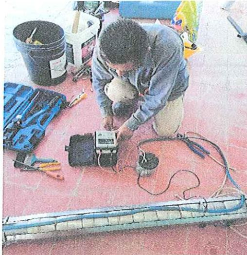
MONTAJE ELECTROMECANICO DE UNA BOMBA SUMERGIBLE 30 HP/440V- 84 MT DE COLUMNA ACERO AL CARBON 4", EN BOMBEO POZO PROFUNDO 8, LOCALIZADO EN LA COL. ALVAREZ DE ESTA CD. IGUALA GRO.
