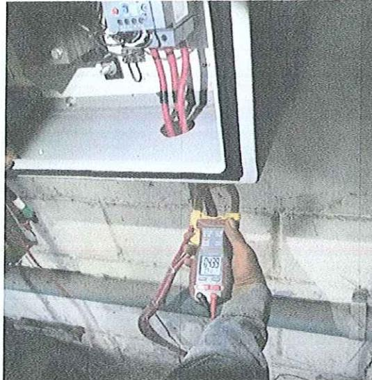
MONTAJE ELECTROMECANICO DE UNA BOMBA SUMERGIBLE 30 HP/440V- 84 MT DE COLUMNA ACERO AL CARBON 4", EN BOMBEO POZO PROFUNDO 8, LOCALIZADO EN LA COL. ALVAREZ DE ESTA CD. IGUALA GRO.
