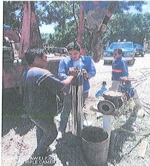
MONTAJE ELECTROMECANICO DE UNA BOMBA SUMERGIBLE 30 HP/440V- 84 MT DE COLUMNA ACERO AL CARBON 4", EN BOMBEO POZO PROFUNDO 8, LOCALIZADO EN LA COL. ALVAREZ DE ESTA CD. IGUALA GRO.
