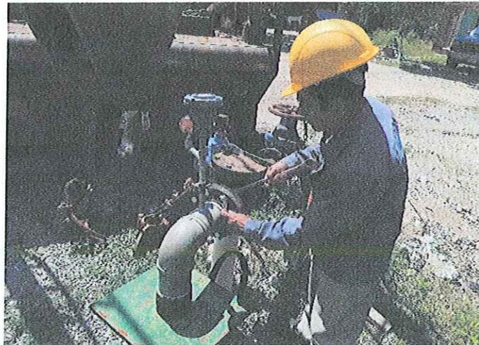
MONTAJE ELECTROMECANICO DE UNA BOMBA SUMERGIBLE 30 HP/440V- 84 MT DE COLUMNA ACERO AL CARBON 4", EN BOMBEO POZO PROFUNDO 8, LOCALIZADO EN LA COL. ALVAREZ DE ESTA CD. IGUALA GRO.
