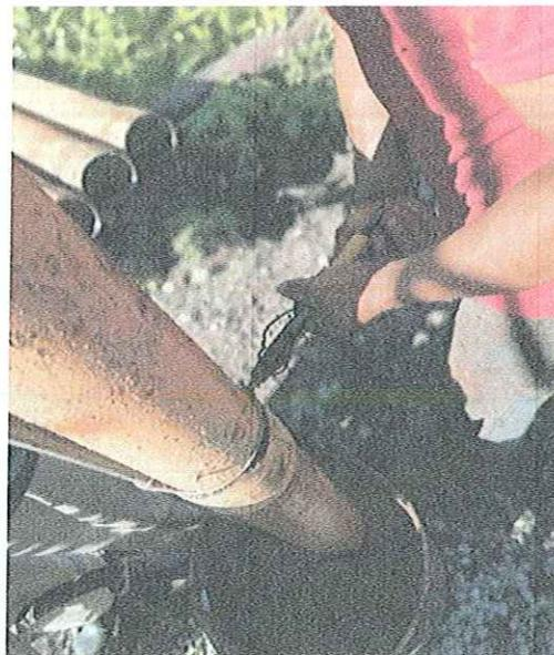
MONTAJE ELECTROMECANICO DE UNA BOMBA SUMERGIBLE 30 HP/440V- 84 MT DE COLUMNA ACERO AL CARBON 4", EN BOMBEO POZO PROFUNDO 8, LOCALIZADO EN LA COL. ALVAREZ DE ESTA CD. IGUALA GRO.
