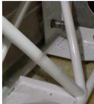
Figure 4: Gusset added to lower plate V2
