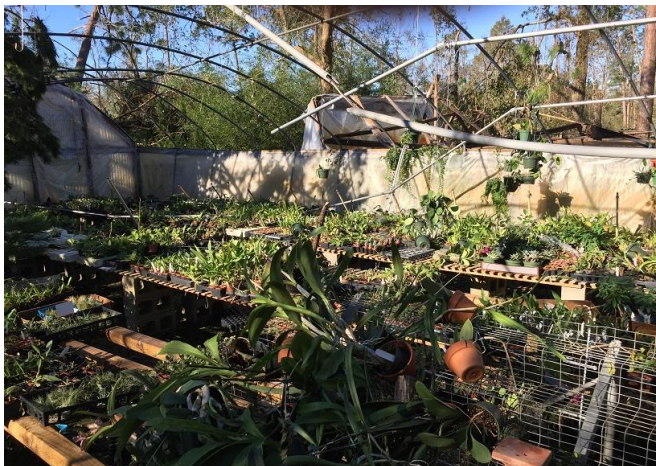
A reminder of the damage a hurricane can do, and this was 55 miles inland!
