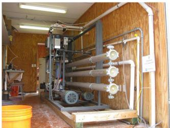
Figure 3 - Osmonics RO Skid 2:1 Configuration
