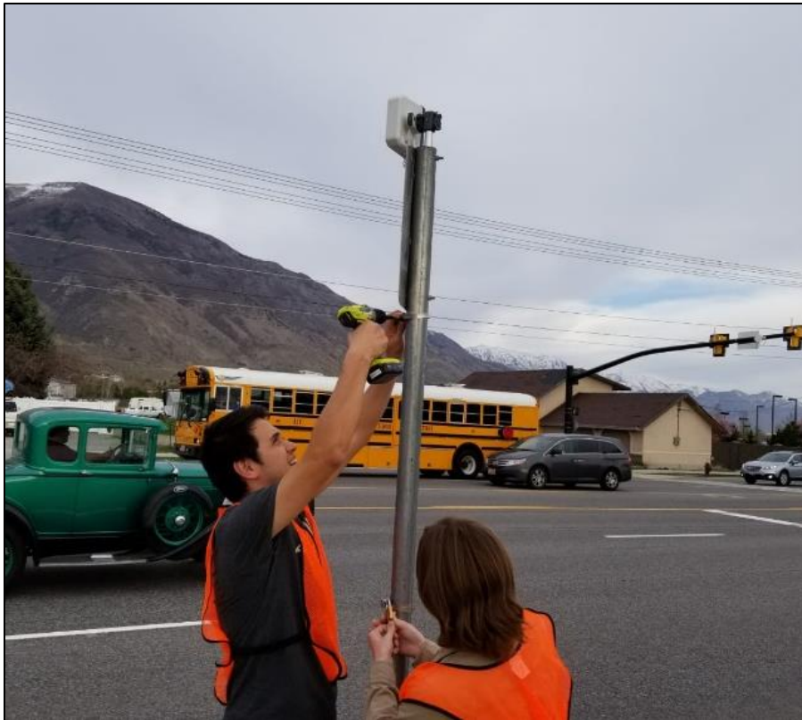
Figure 3.2 Research Assistants Mounting a COUNTCam2 Camera
