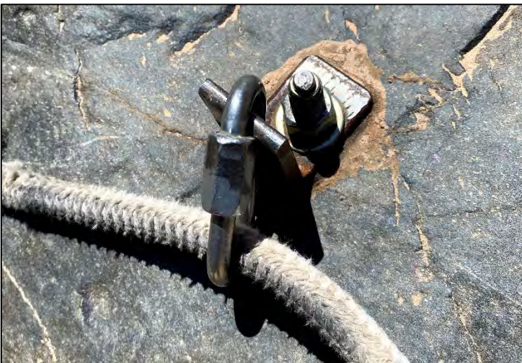
Hardware for connecting a rope handhold on a steep incline at Grand Canyon National Park.
