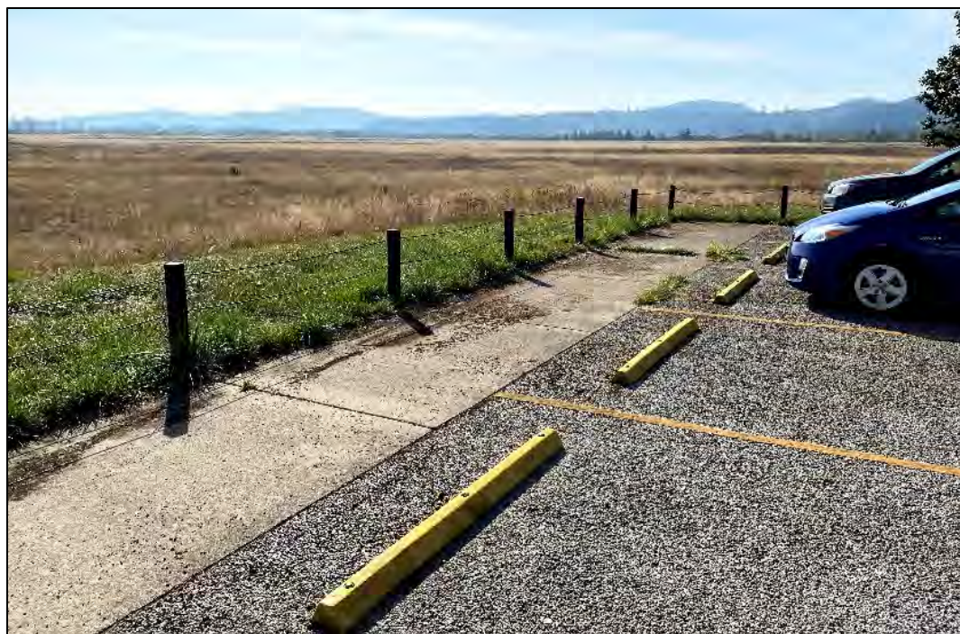
An example of cable fencing and wheel stops at the Meadowlark Prairie parking area near Eugene (example shown includes permeable concrete pavement – gravel is recommended for the Fisher Preserve)
