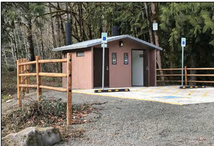
A "Forest Service style" concrete pre-fabricated vault toilet at the McKenzie River Trust's Finn Rock Reach boat ramp Reach
