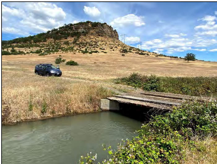
Driveway access and irrigation canal bridge with Pompadour Bluff in the background
