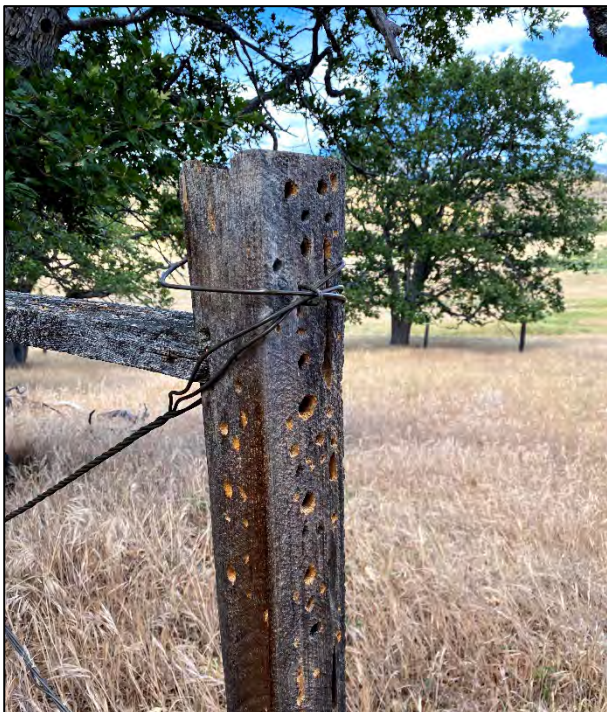
An existing fence post at the Fisher Preserve (shown above) with Acorn Woodpecker workings could serve as inspiration for unique wayfinding posts that could be fabricated using rot-resistant rough-cut juniper, drilled to resemble a granary tree.
