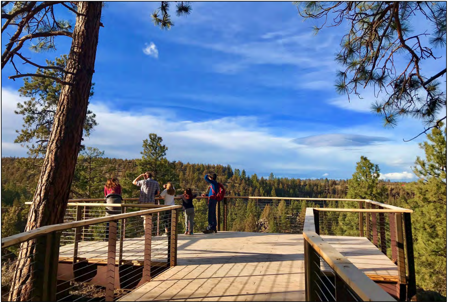
A viewing platform at the end of the trail on the steep cliffs overlooking the Deschutes River at Riley Ranch in Bend (constructed with rough-cut juniper framing and decking)
