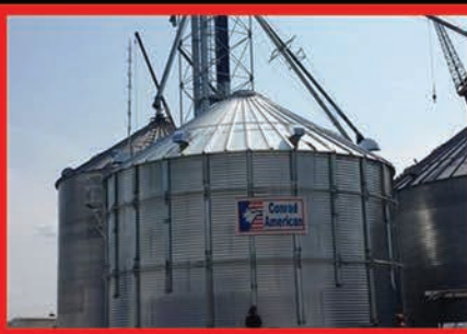
Grain Bin Construction and Remodeling
