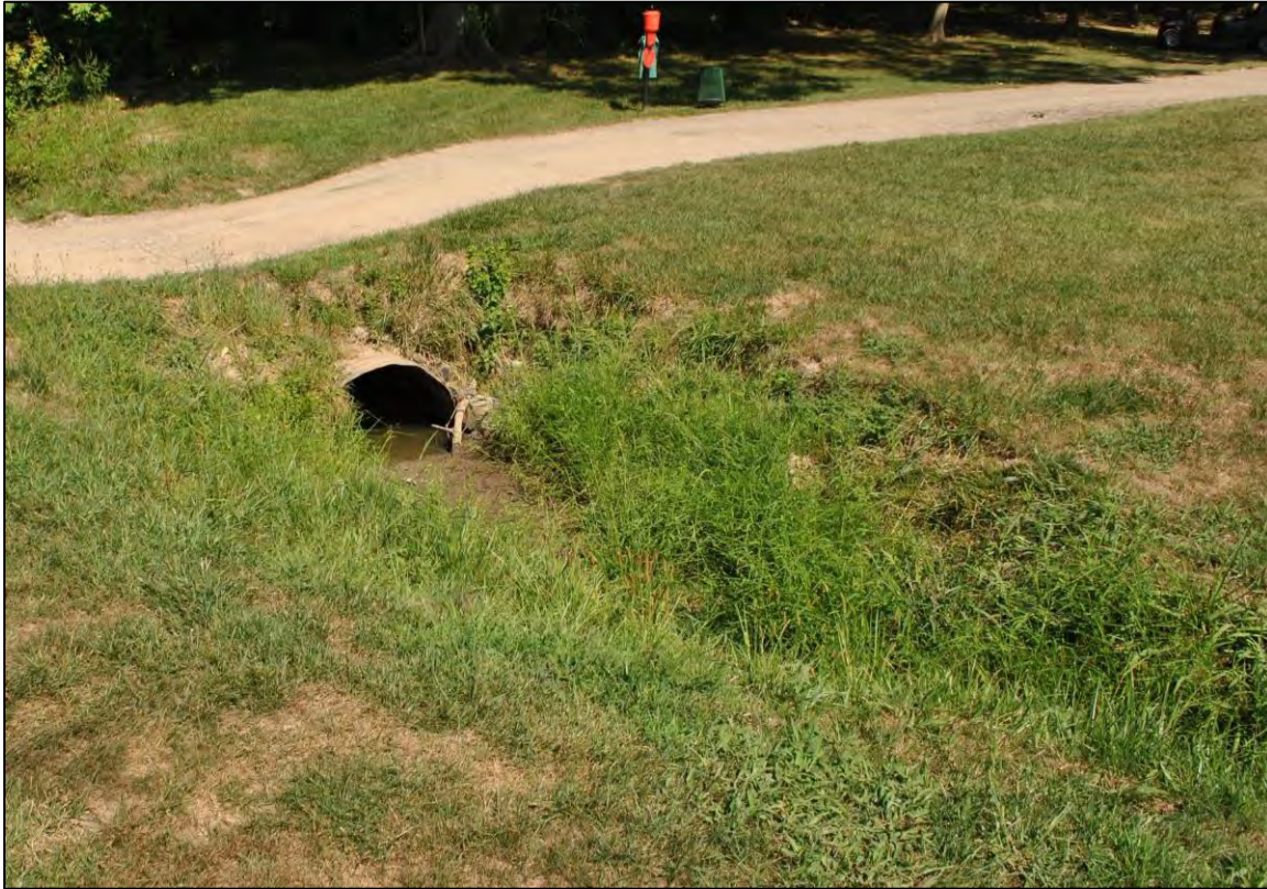
Figure 4-2: Culvert beneath Cart Path downstream of 7 th Tee
