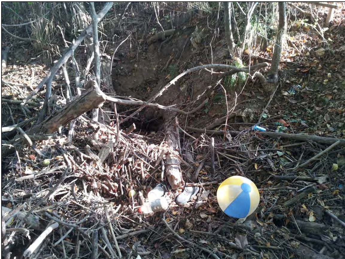
Figure 4-1: Upstream culvert entrance beneath Pro Tour Drive near 10 th Fairway Drive
