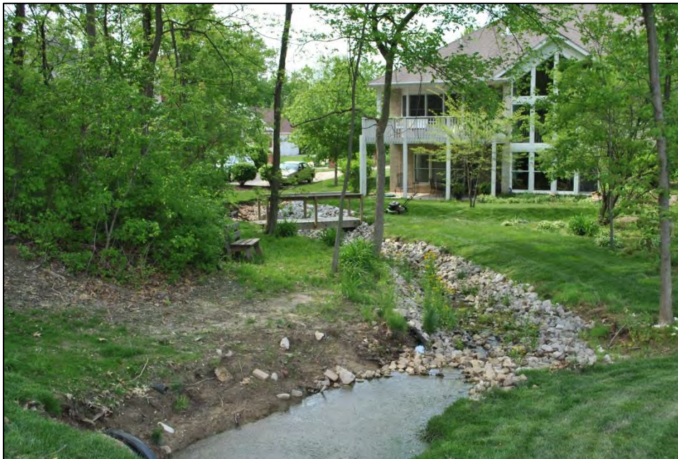
Figure 4-9: Area Downstream of 8th Hole
