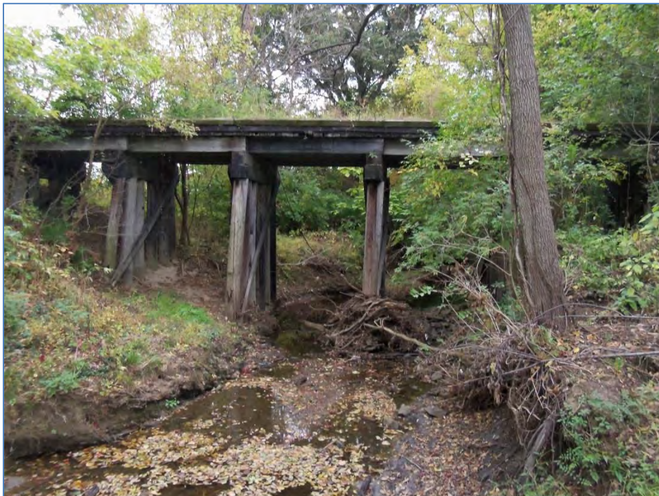
Figure 4-20: Railroad Trestle Downstream of Development
