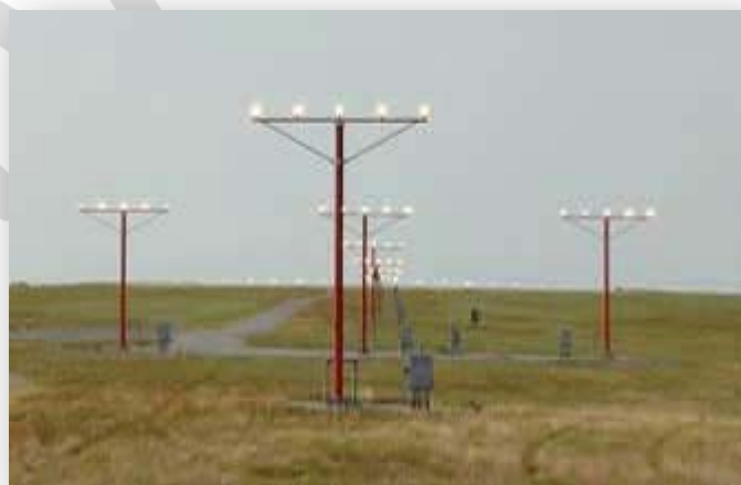
Figure 2-7 MASLR RW 14 Approach (picture not of ASH)
