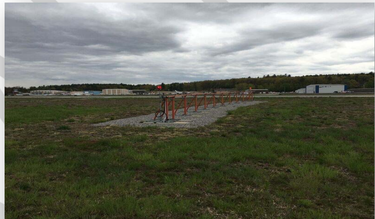
Figure 2-9 End Fire Glideslope Runway 14 End
