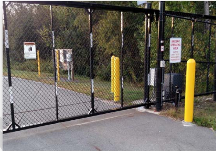
Figure 2-11 Perimeter Fencing- Gate 15
