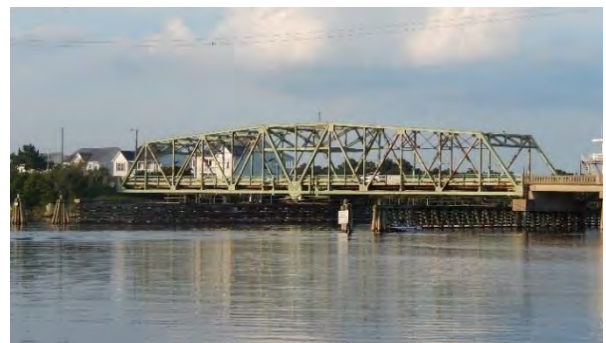
Topsail Island Bridge No. 16 (Pender County)
