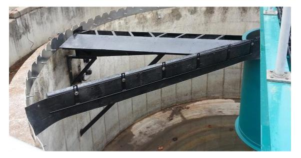
The full radius scum trough features a much larger collection area, causing more sludge to be removed with each pass. Also our trough features less components and a more straight forward design compared to most collection mechanisms making maintenance easy and inexpensive. Fab Tech has extensive experience repairing and upgrading circular clarification units, all installation is performed by our trained field service personnel.
