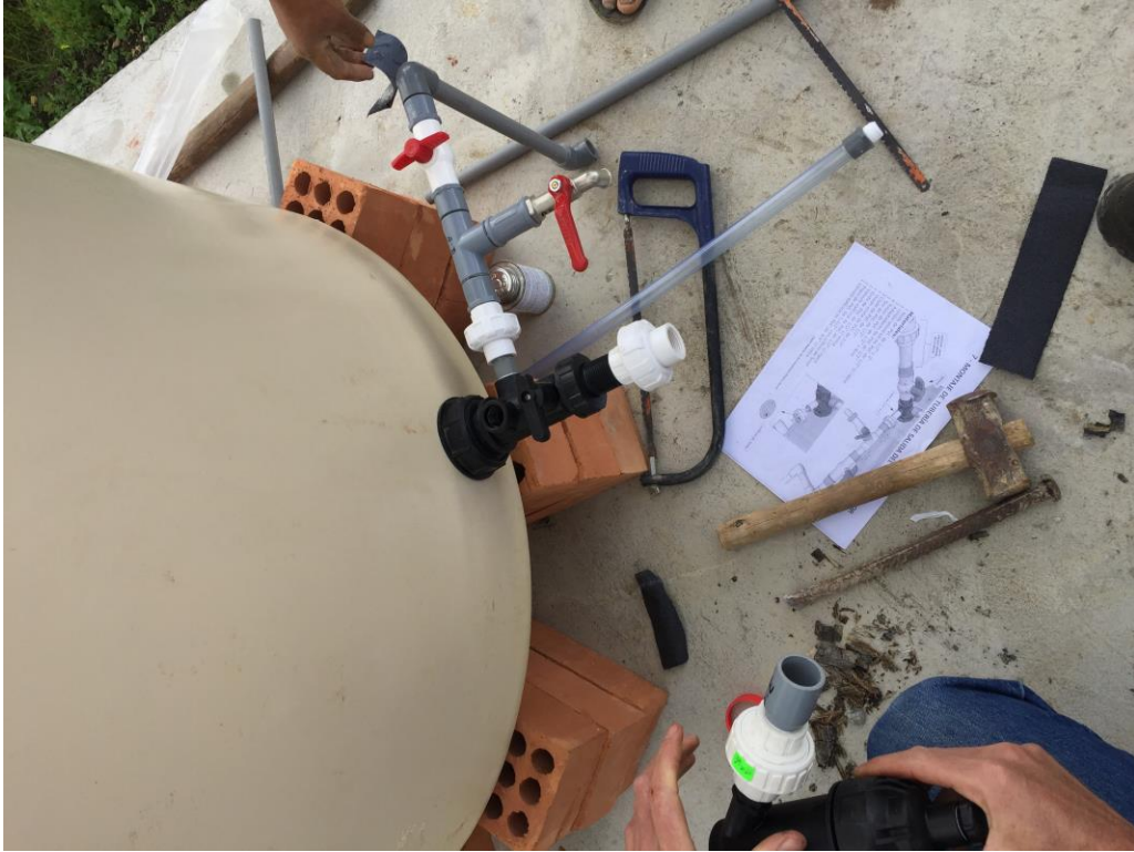
Setting up a 600-liter drip chlorine system to serve Shipata's reservoir.
