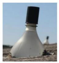
Take a 2l clear clean plastic bottle fill it 1/2 with water. Add 2 cupfuls' of bleach to stop Algae from growing. Top up bottle with water to rim & put on cap. The lamps work best with a black cap. Make a hole in roof. Push bottle through hole, cap 1st. Seal hole with polyester resin.
