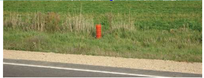
Figure 5: Tile vent installed at field edge.
