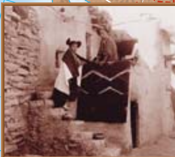
Pueblos, built of sun-dried brick, or adobe, were characteristic dwellings of the Southwest.
