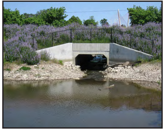
Box culvert under Goodpasture Island Road
