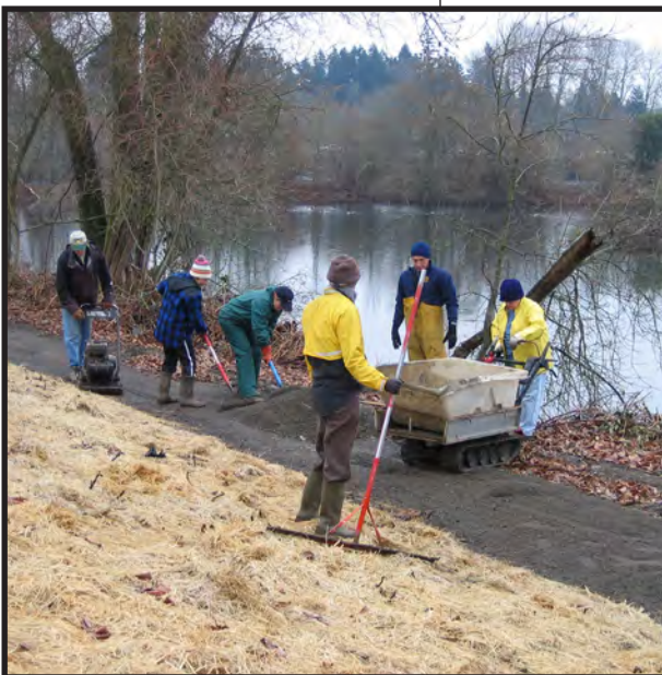
Volunteers constructing the north trail
