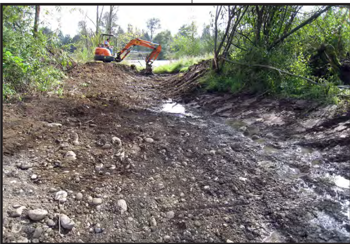
Excavation of the northernmost channel near the Dedrick Slough outlet
