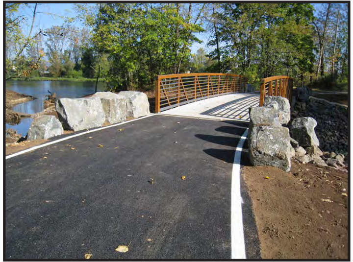
Bridge over Heron Slough
