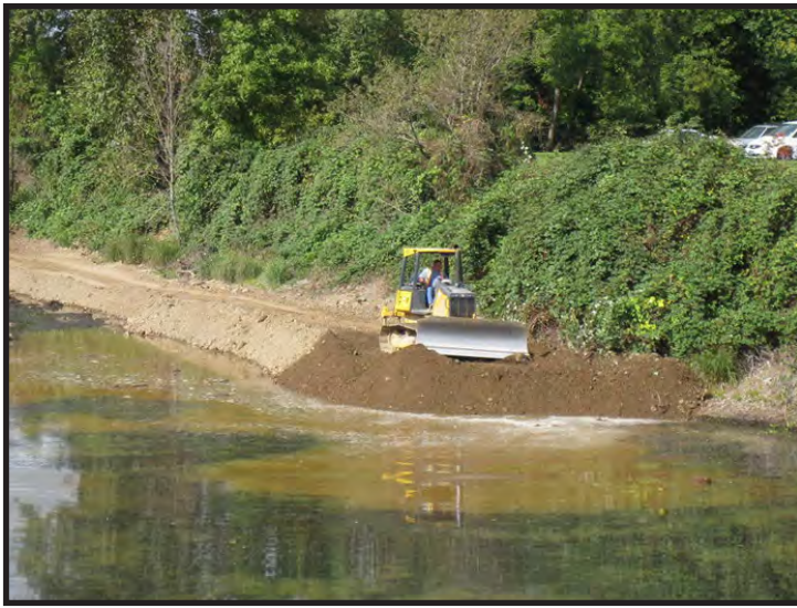
Grading riparian bench
