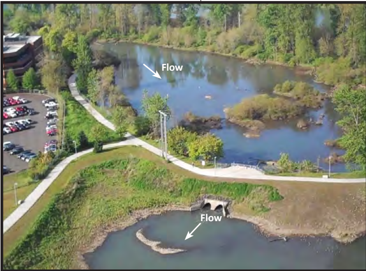
Gated culvert under the levee and multi-use path
