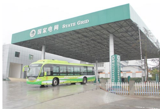
Figure 5: The world's first ultrafast charging station in Chongqing, 2012 69
