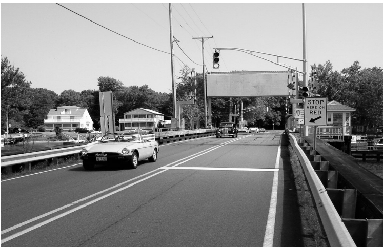
(above) Tour crossing Green Bank Draw Bridge
