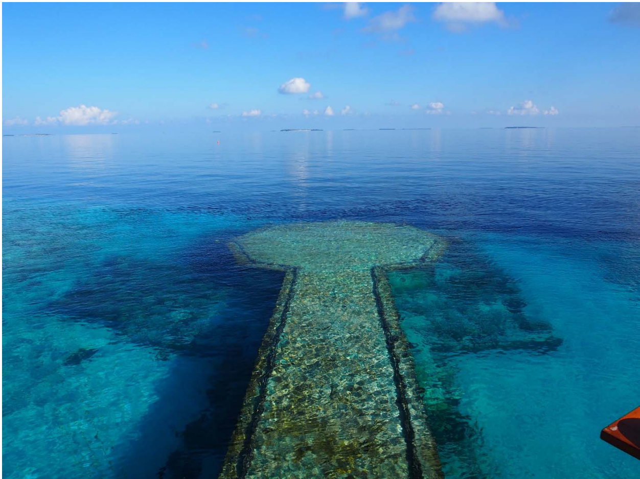
Fig. 1. SEA photographed from the deck. The roof of the long walkway and octagonal restaurant are situated within a sandy area in a cut between the reef. A submerged platform surrounds the structure. The edge of the drop-off is about 3-5 m from the front of the restaurant. The roof is in 1-3 m depth (depending on tide) and the cement platform ranges from 3-5 m depth.
