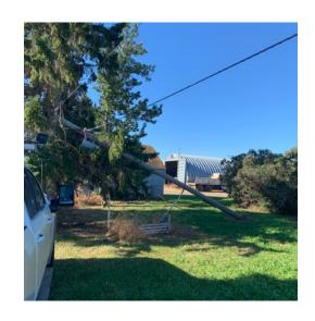
Identify Potential Hazards: Familiarize yourself and your team with the location of power poles and lines near your fields. Take note of any low-hanging lines or damaged poles that may pose a risk during seeding operations. If you see a broken pole or there are downed lines, do not try and touch the lines to move them. Call your maintenance provider. Downed lines have the potential to be live and can be deadly.
