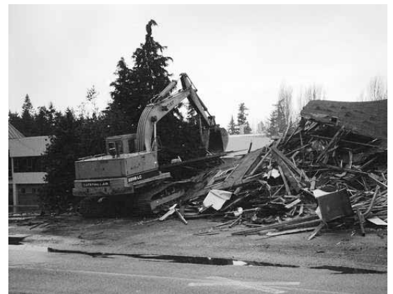
Historical Huts Demolished 2ND WW till 1994
