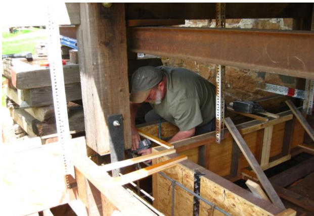
Steve Winchel at work on the foundation.
