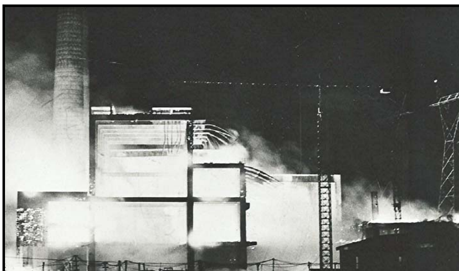
Figure 3 – Ap Lie Chau Power Station Fire
