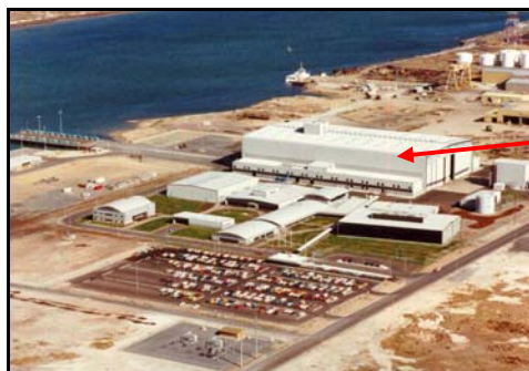
The ASC Adelaide facility
