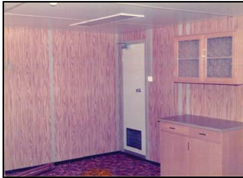
Fire doors and bulkheads
