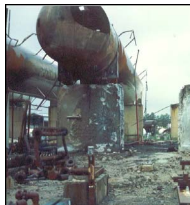
The destroyed Boral facility
