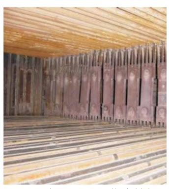
Fig-2: Support plates separating two assemblies of coiled tubes.
