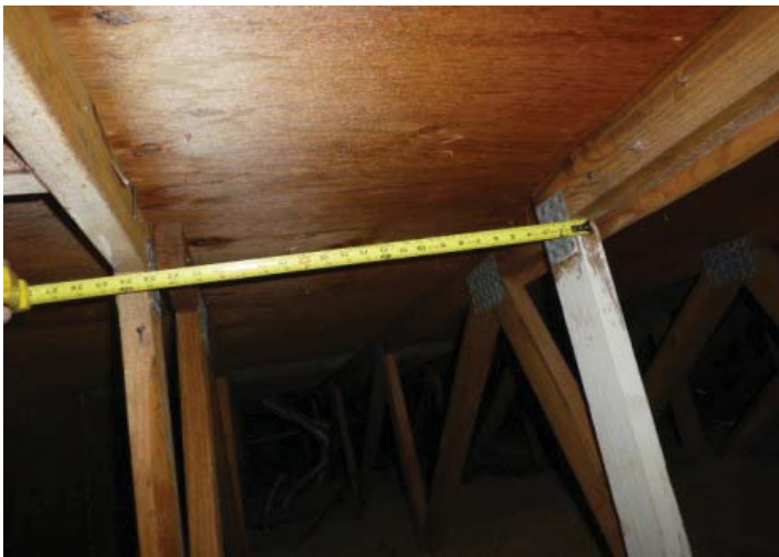
TRUSS/RAFTER SPACING
