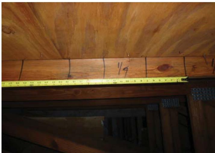
#3 ROOF DECK ATTACHMENT 6" X 6" NAIL SPACING
