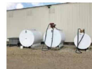
(2) 1000 gallon diesel fuel tanks w/pump
