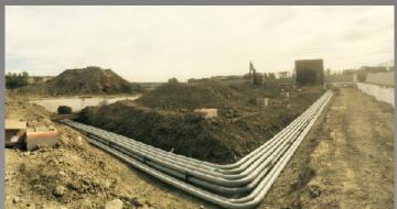
Complete electrical base building build out of a 29 unit commercial strip mall. Starting with a clean slate we began with the underground conduits and conductors and worked our way to the top finishing with the roof top units. This project required a 2400 amp service as well as a complete fire alarm system.
